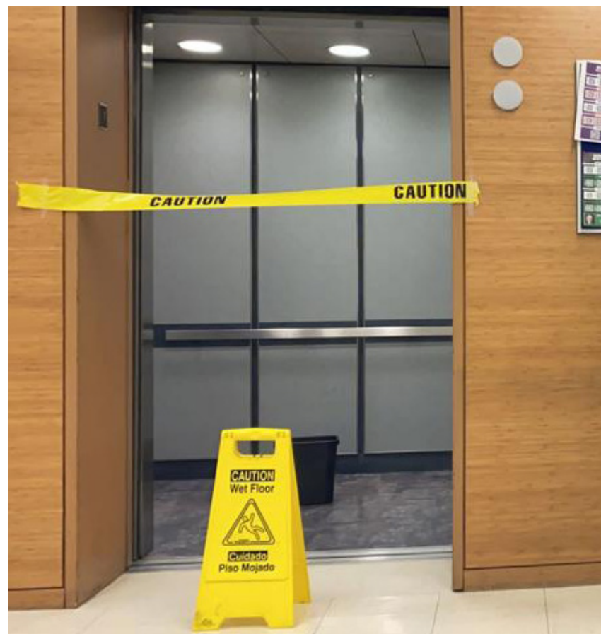
One of Stanton Hall's elevators. 2 of 3 were out of service.
