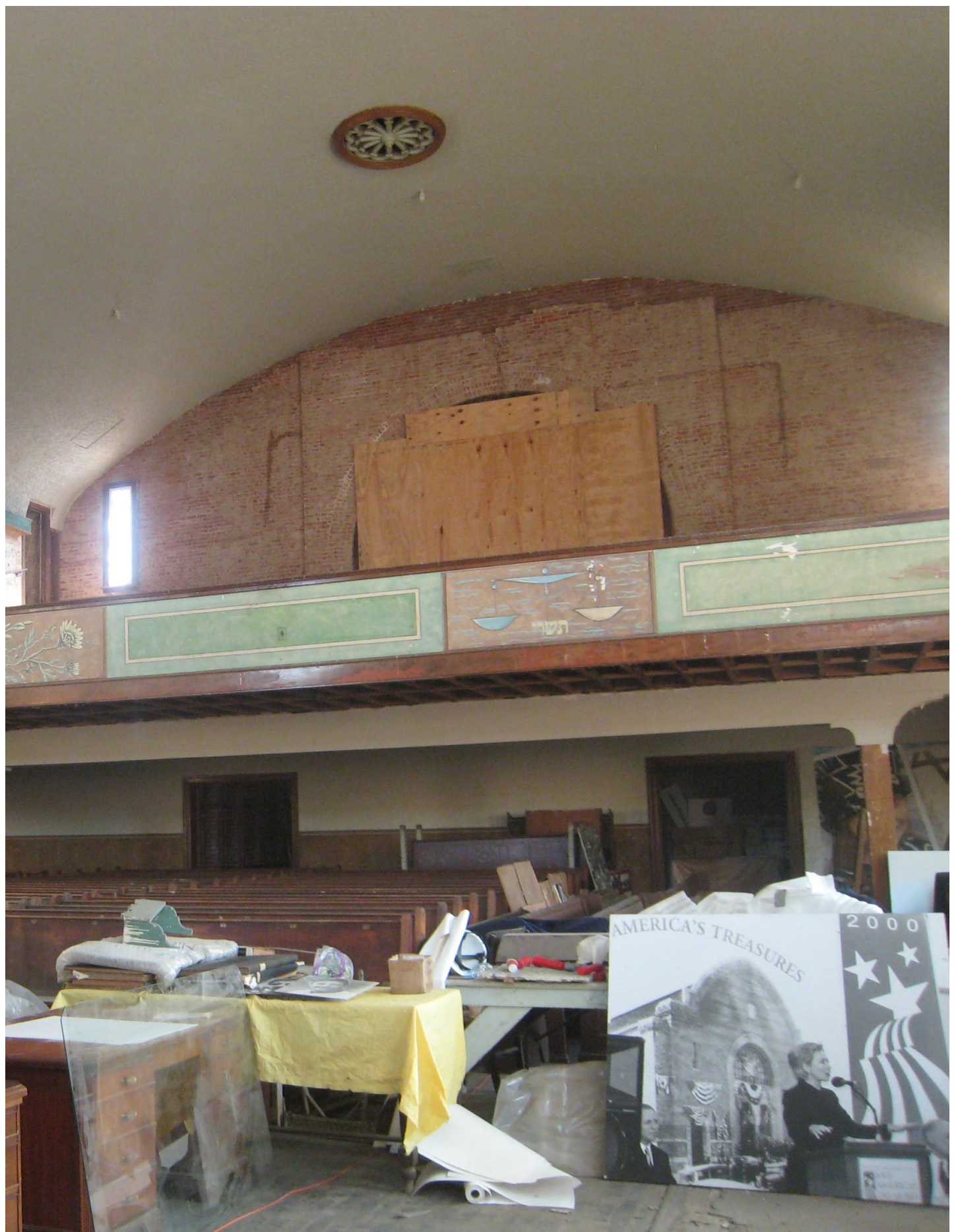
The Breed Street Shul in Los Angeles, California, which has deteriorated over time.
